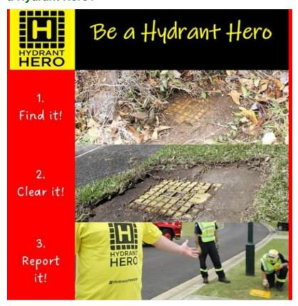
There have been numerous incidents throughout the State where firefighters have been unable to access the nearest hydrant in an emergency due to it being poorly marked, obstructed by parked cars, mud or debris, or over-grown vegetation. Poorly maintained or unusable hydrants result in critical time being lost while firefighters clear the hydrant or search for and access another hydrant further from the fire.
