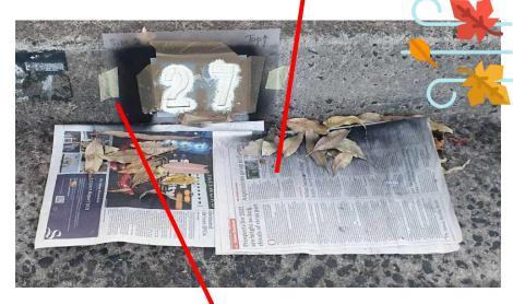
Without protecting the area, it may cause overspray or damage the environment
